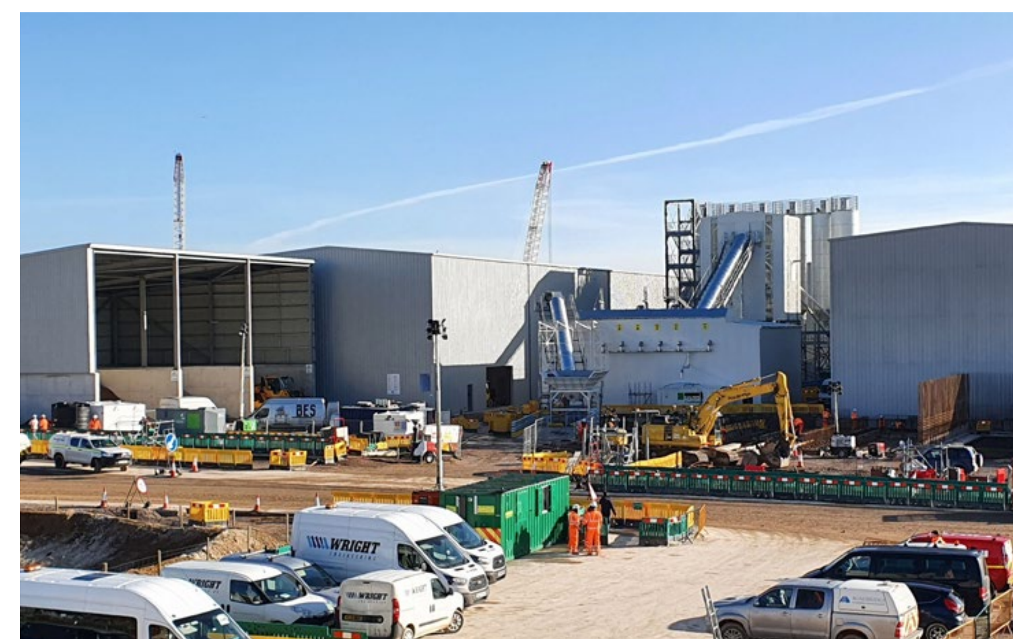
Pre-cast concrete factories for the tunnel lining
