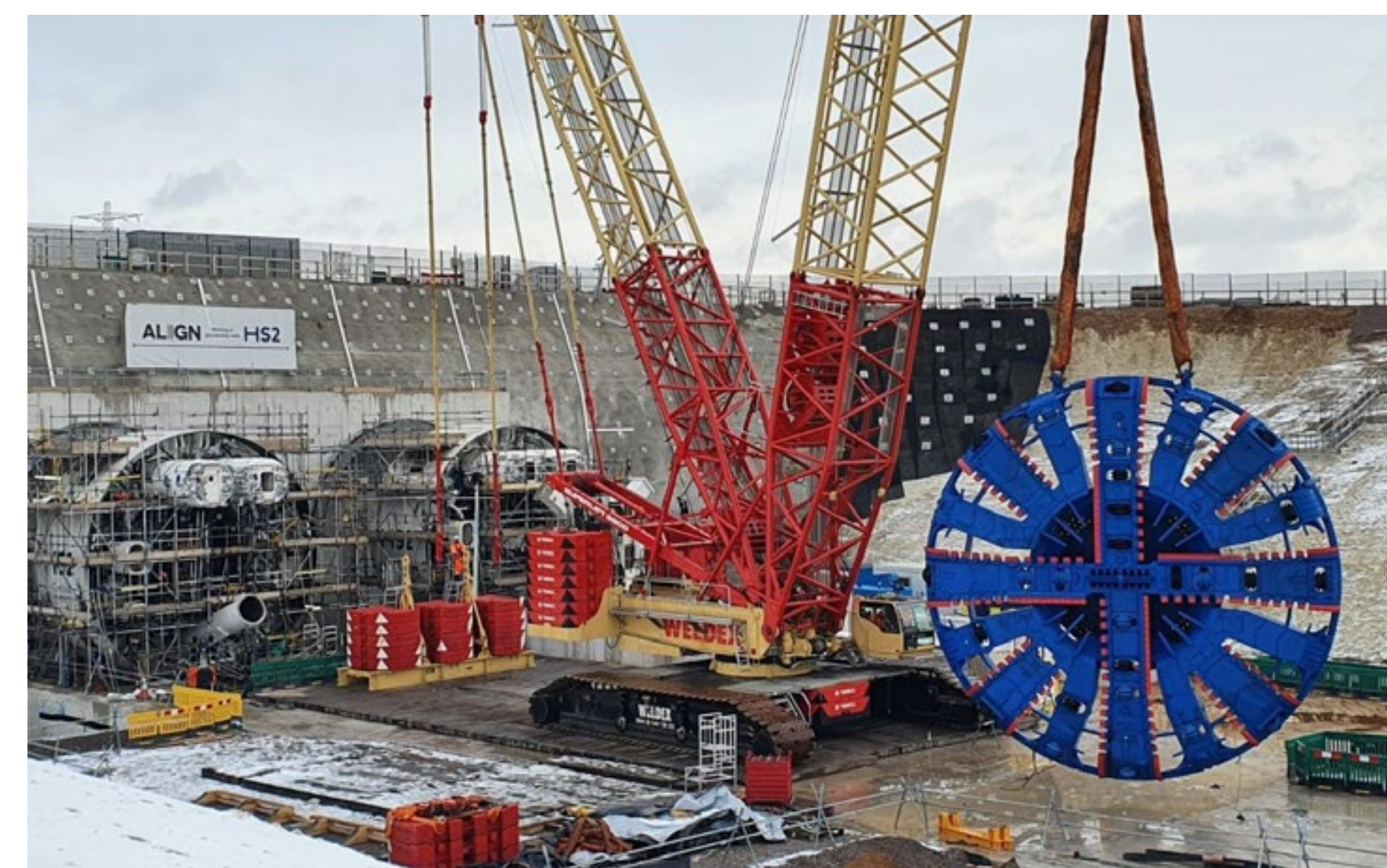
Tunnel Boring Machine assembly at the South Portal
